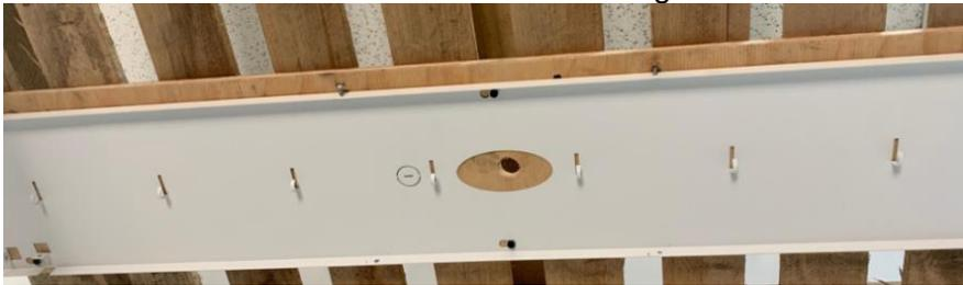
3. Position the fixture parallel to the surface mount kit and insert the wires through the center opening.
